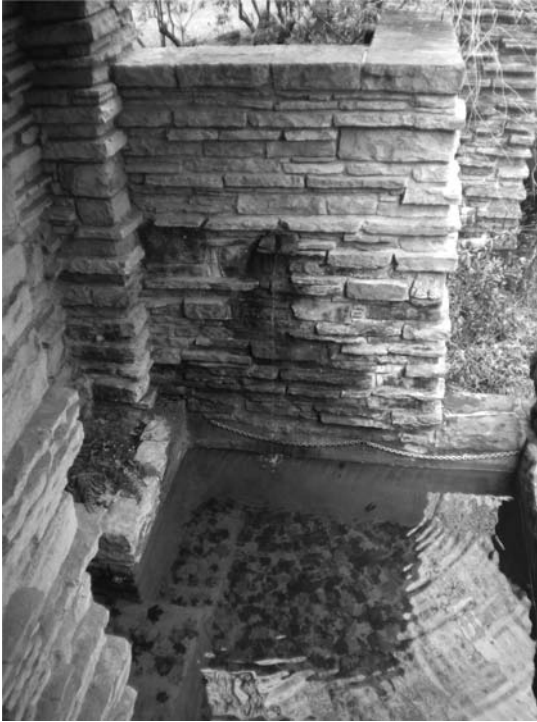
Figure 8. Entrance bath Fallingwater
