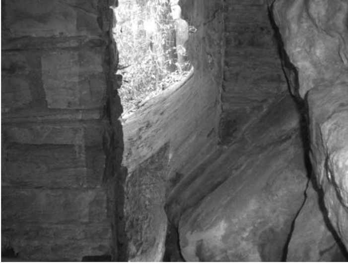
Figure 4. Interior basement living rock w masonry, Fallingwater
