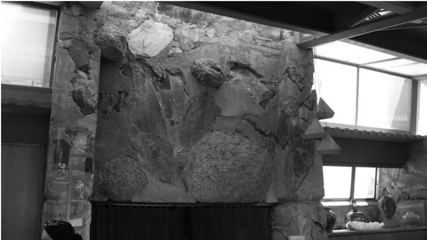
Figure 10. Taliesin West, chimney w embedded living rock, main house
